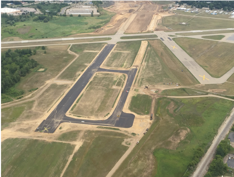
Aerial view of runway work in progress 2016-2017
