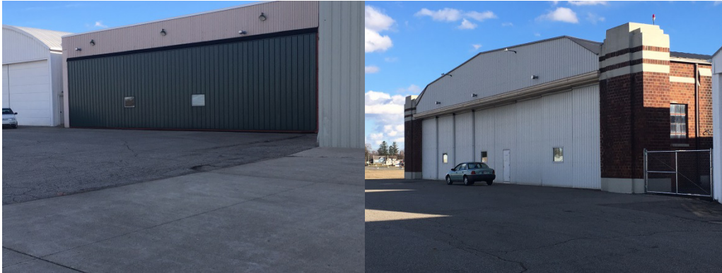
Hangar #204 Jackson County Airport
