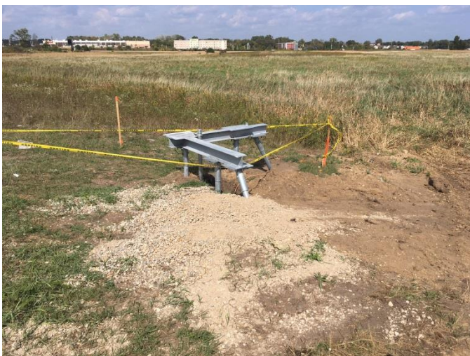
(5) Piles connected to a bracket
