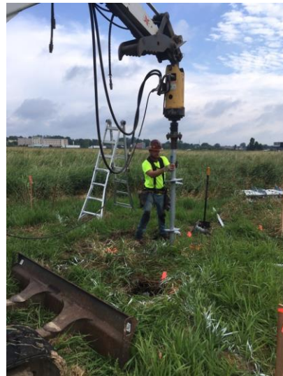
Drilling the piles
